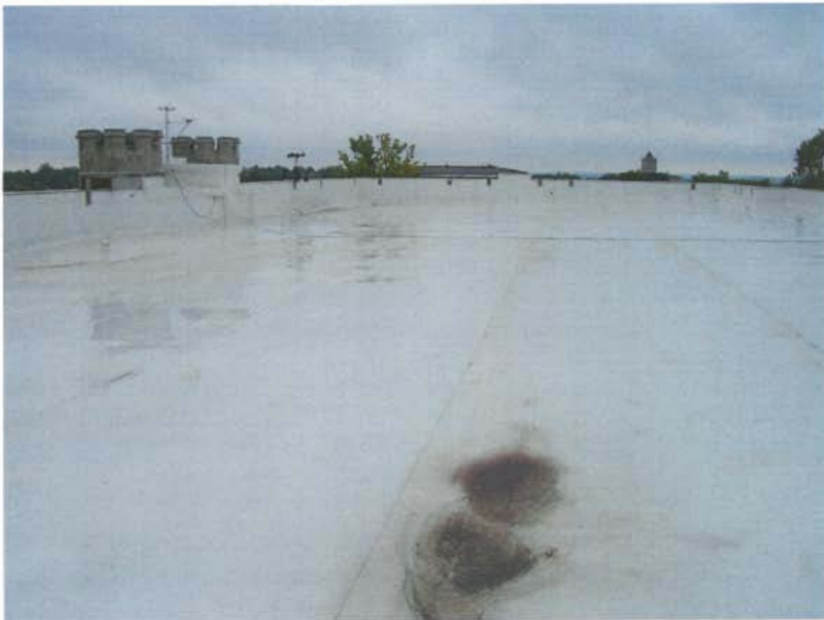
Photo #7: Roof looking south. Membrane appears to be in good shape and has ample slope for drainage.
